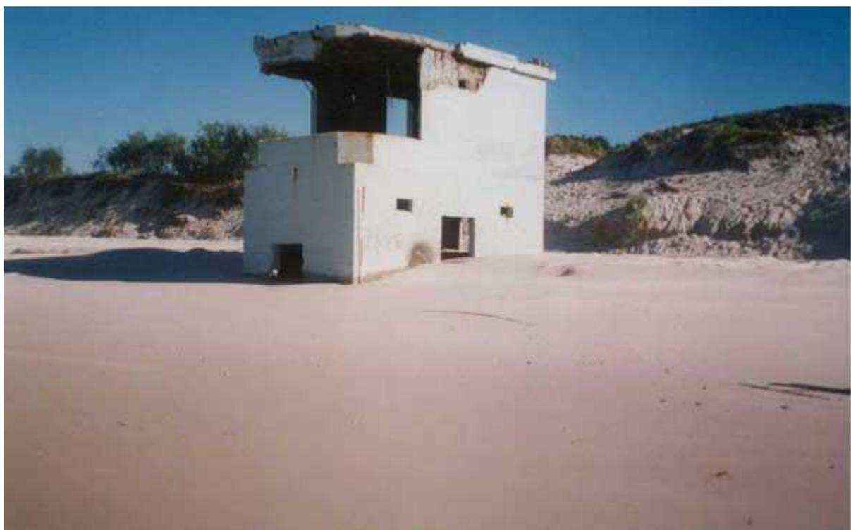
**Photo 2.** Long-term erosion of the beach on the spit at the northern end of Bribie Island, SE Qld. This WWII gun bunker was originally built behind the beach on the foredune, which now sits behind the bunker. (Photo by J. Lester).
